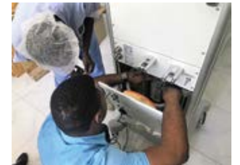
Dr. Stanley Loriston, anesthesiologist, finalizes installation of the universal anesthesia machine at Serving Sante
