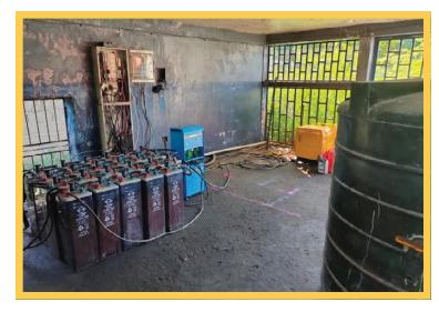
room, and (4) re-wiring the hospital's electrical distribution system to create two load centers. These improvements will reduce the strain on the battery and solar systems and in turn, strengthen the overall system.
