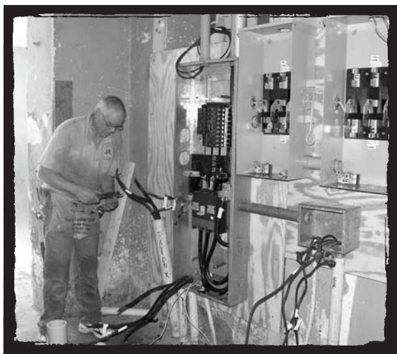
Gary LaClaire installs new electrical panels.
